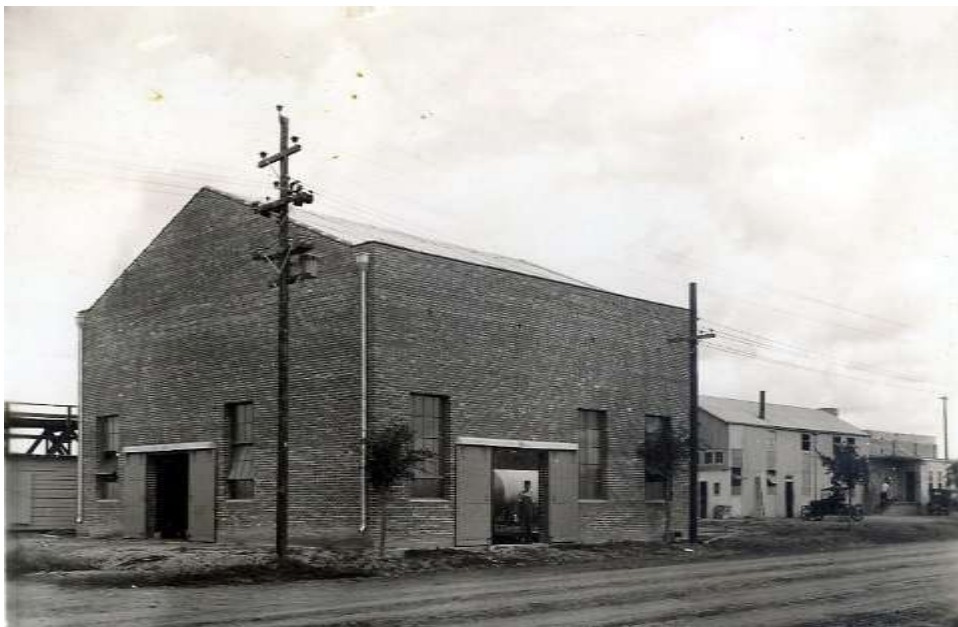
Figure 4. Power house, Central Power and Light Company; Crystal City, TX (Photo courtesy of Joe Taylor).
