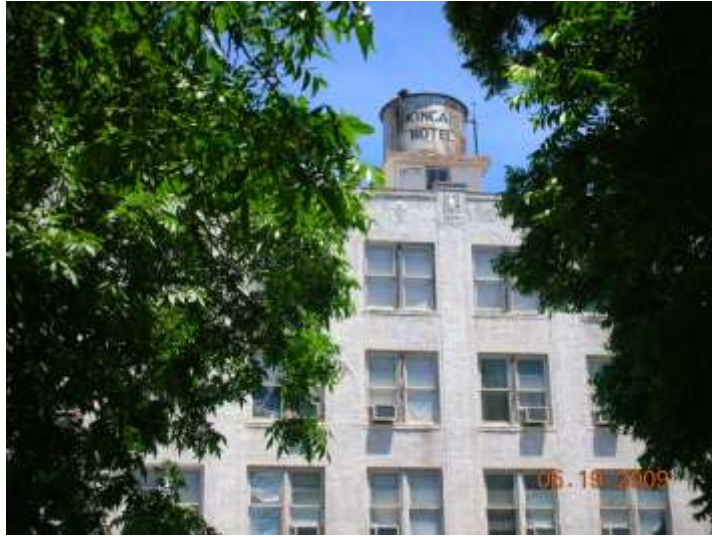
Figure 18. Kincaid Hotel, as seen today Uvalde, TX.
